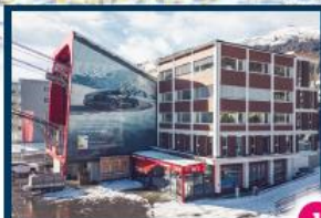
Race Office Talstation Jakobshorn
